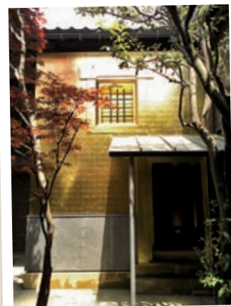
The "Golden Storehouse" features a gilded platinum-leaf exterior and 24 kt gold-leaf interior.
